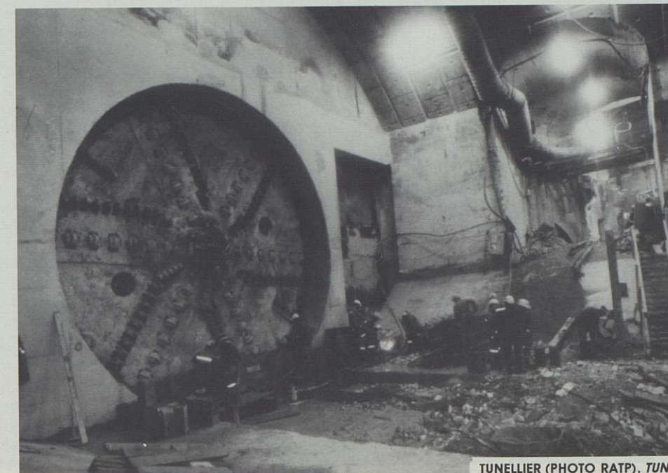
TUNELLIER (PHOTO RATP), TUNNELING MACHINE
